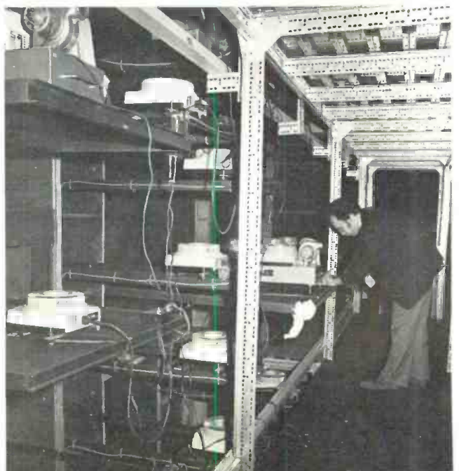
Figure 6. Backstage at the Mill in the projection area. Note the perforated steel platforms on which the projectors are mounted.
