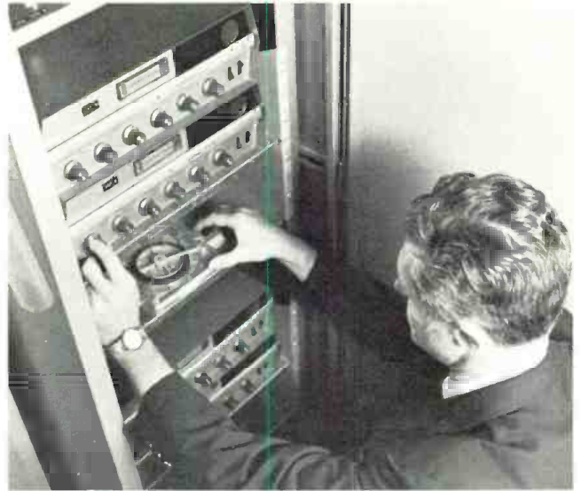
Figure 5. The author is seen starting one of four amplifiers/tape decks. Each amplifier has a monitor speaker which can be cut off by the switch below it. During the check-out period at down time, test levels are set.
